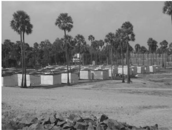
Figure 7: Housing units of jute-bitumen corrugated sheets constructed on the wrong side of the highway remained unoccupied, because of the hazard of crossing the road while coming from and going to the coast. Source: (Murty, Jain, Sheth, Jaiswal, & Dash, 2006).
