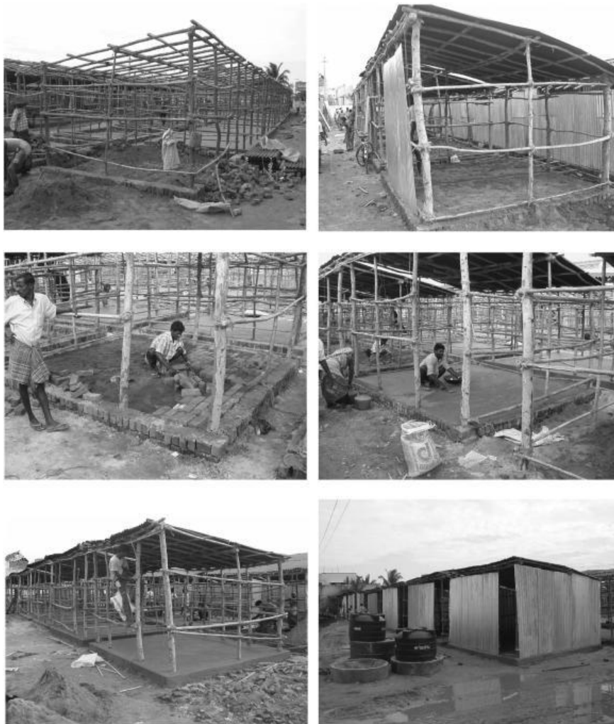
Figure 6: Temporary shelters built by Government using GI corrugated sheets, wooden ballies, nails brick to level up the ground at Tamil Nadu. Source: (Murty, Jain, Sheth, Jaiswal, & Dash, 2006).
